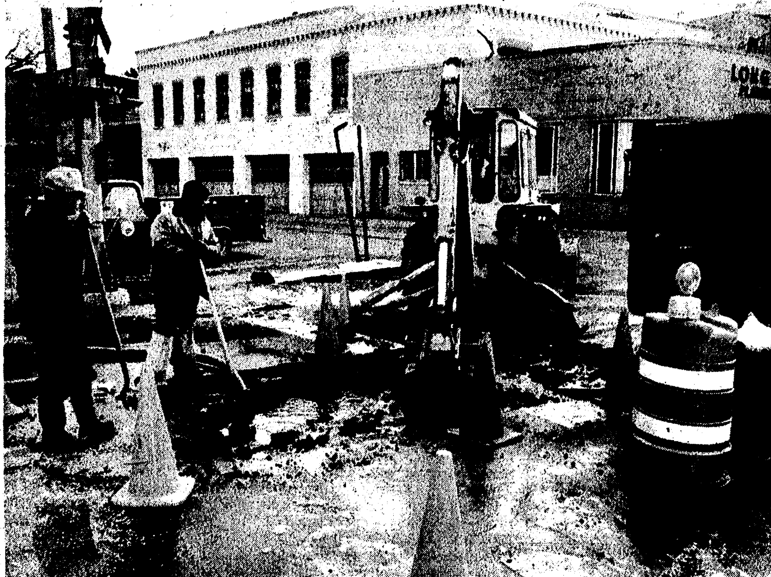
A WATER MAIN BROKE on Main St. over the weekend, forcing a detour of traffic for most of the day. Village employees worked into the night to stop the break, which had water gushing onto Main St. According to utilities superintendent Bud Hafner, the pipe involved was probably some of the original pipe in the village, which was installed before the turn of the century. Three water lines have broken in the last week, Hafner said.
